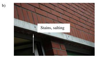
Fig. 1. Setting of window in the three-layer wall; a) view the installed windows from the inside b) the method of attaching aluminium canopies above the windows
